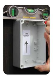
Offer the back of the eoMINI up to the installation location; make sure the surface is flat and level. Level the eoMINI back and mark the position of the 4 holes
