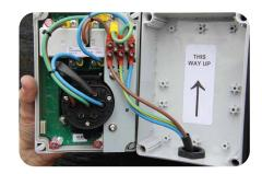
Offer up the eoMINI front section and connect the power cables as shown
